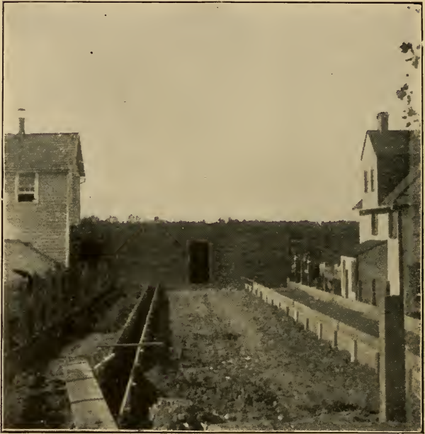
26.—Constructing house twenty-four feet wide; second step, making beds and walks
